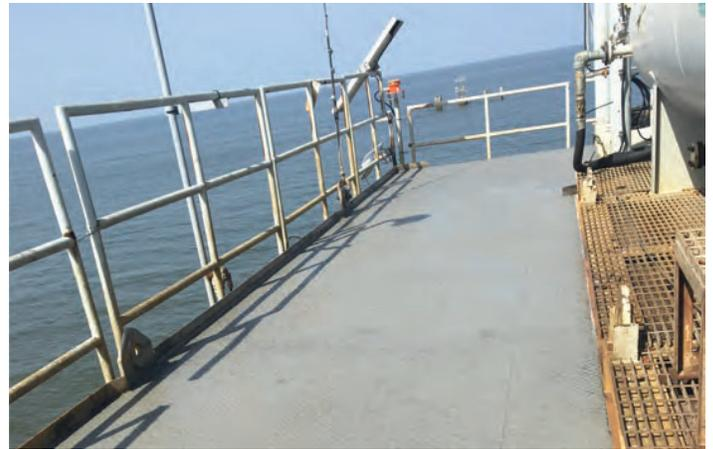
Blasting/grinding was not an option for this location. CRS allowed the applicators to protect the substrate by just power washing and de-greasing before applying CRS. C2M was applied as a topcoat after drying.
